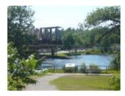
Big Chute Marine Railway is a boat lift at Lock 44 of the Trent-Severn Waterway in Ontario, Canada. It works on an inclined plane to carry boats in a cradle (without a filled tank) over a change of height of about 60 feet (18 m). It is the only marine railway of its kind in North America still in use.
