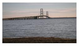
Opened on November 1, 1957, the Mackinac Bridge was the longest suspension bridge in the world. It is still the longest suspension bridge in the western hemisphere. Although the 3,800 foot center span is slightly shorter than the center span of the Golden Gate Bridge, the total length of the Mackinac Bridge is 26,372 feet. The length of the suspension bridge (including anchorages) is 8,614 feet.
