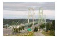
The Tacoma Narrows bridge is a pair of twin suspension bridges that represent the second attempt to span the Tacoma Narrows strait of Puget Sound in northwest Washington State. The original bridge, which opened in 1940, catastrophically failed during high winds later that same year.
