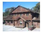
Constructed in 1909-10, this is the only remaining structural log railroad depot in the country. Built for the Atchison, Topeka and Santa Fe Railroad, it helped establish the rustic nature of the Grand Canyon by being the first building the railway passengers encountered upon arriving.
